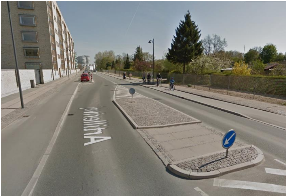
Example of partial road closure (no entry, bicycle excepted) with raised threshold at entry to local street, Brunswick, Victoria.
