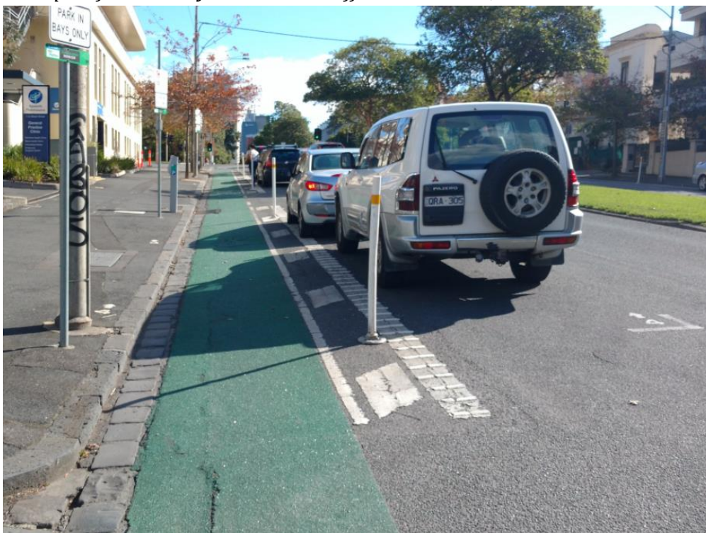
Example of low cost cycle track or 'buffered bike lane', Melbourne CBD
